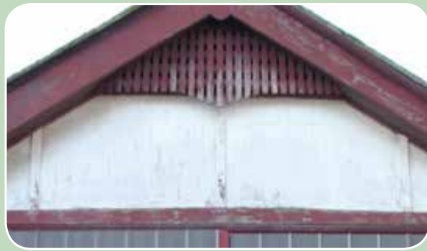
... and in the gable end of a garage
