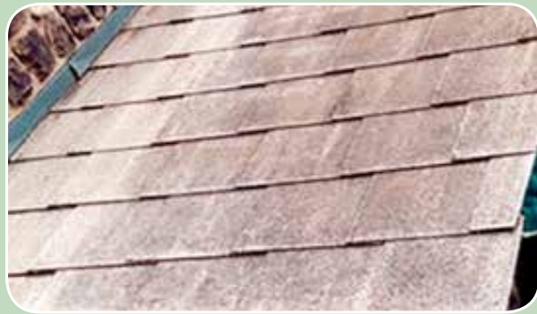
Asbestos cement shingles
