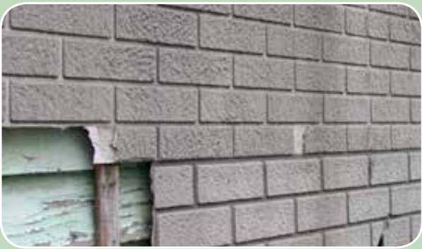
Asbestos cement 'brick' cladding
