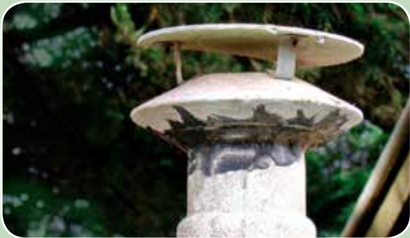
Asbestos cement flue and cowl
