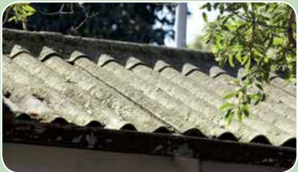
Asbestos cement corrugated roofing
