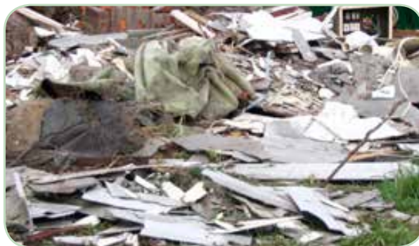
Broken asbestos cement materials from a demolition
